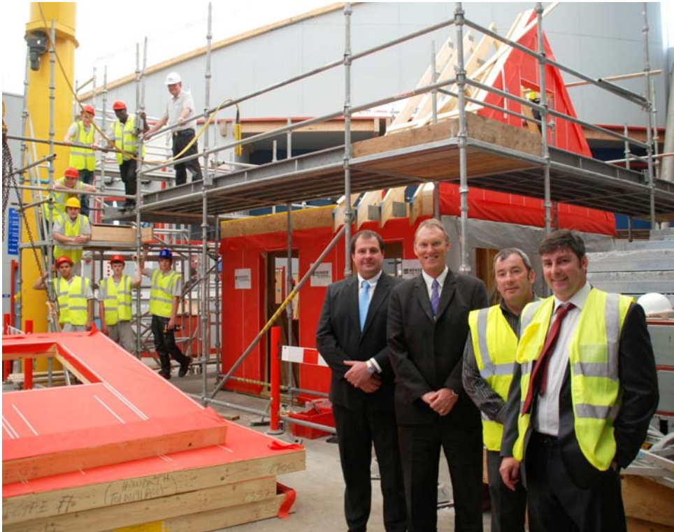
The house goes up: CRC principal Rick Dearing and Construction Academy head John Malone with Jason Dorks and Gary Coulson from Howarth Timber
